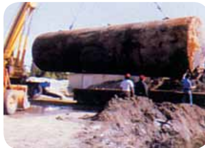
Underground tank removal and on-site demolition.
